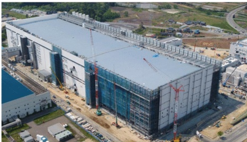
K1 facility (under construction)
